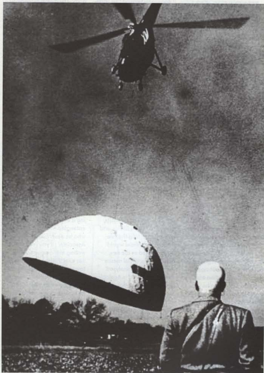
Buckminster Fuller supervising the first airlift delivery of U.S. Marine Corps shelter in 1954.
