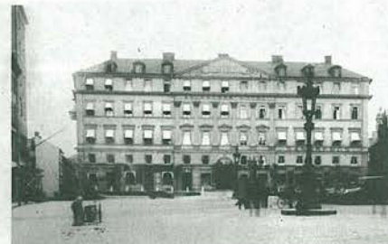
Demolishing the past.
